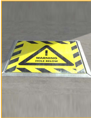
Mark openings with permanent markings.
