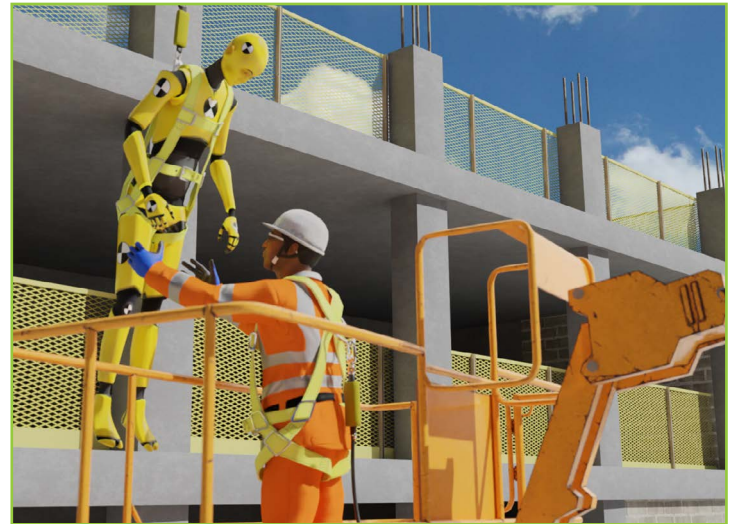
Rescue drills must be carried out prior to work starting.
