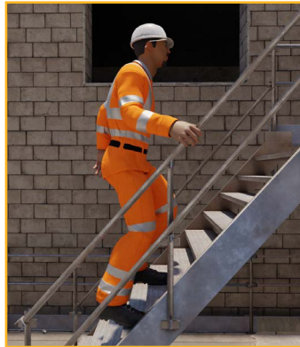
Staircases must have a handrail system in place.
