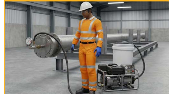
Pipe pressure testing restraints.
